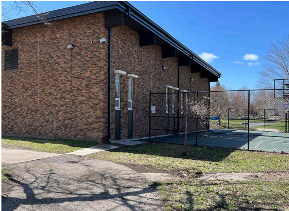
Rec center and basketball courts from the east April 2023
