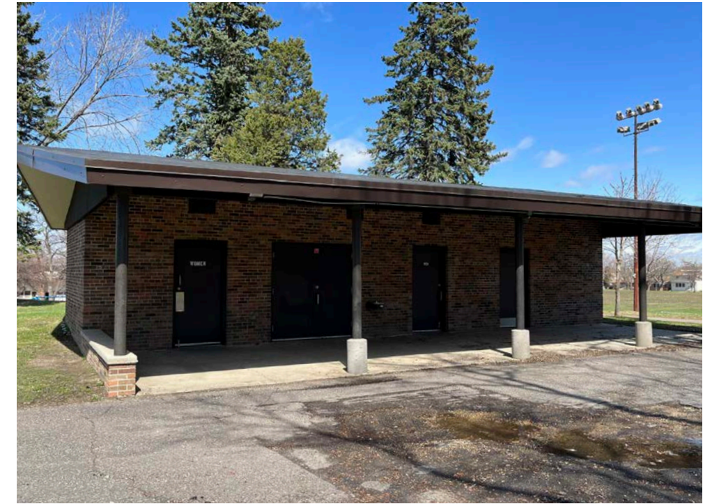
Restroom building at the center of the park April 2023
