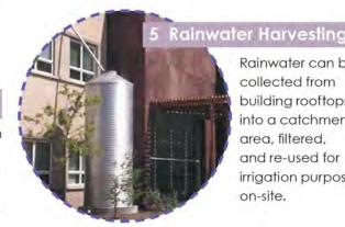
Rainwater can be collected from building rooftops into a catchment area, filtered, and re-used for irrigation purposes on-site.
