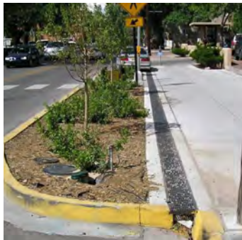
Green Bump-Outs. Source: National Association of City Transportation Officials
