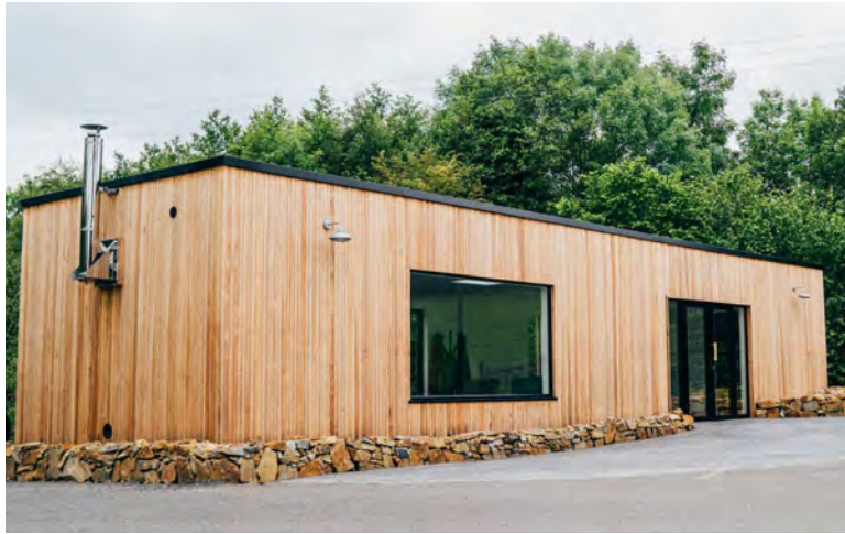
Example of an upgraded temporary warming house. Source: KES Group
