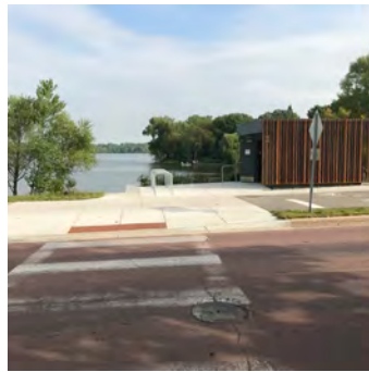
Cedar Lake Parkway crossing at Cedar Lake South Beach
