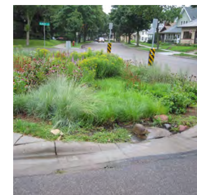
Rain Garden Planting
