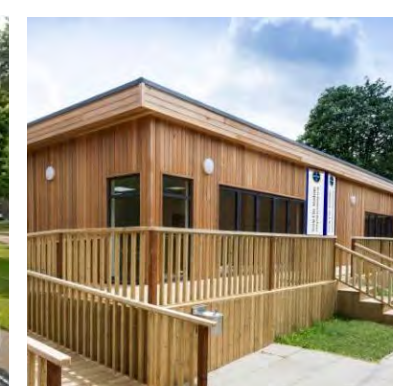
Temporary Warming House
