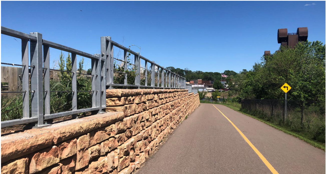
Figure 7 – Prefabricated Modular Block Wall Example
