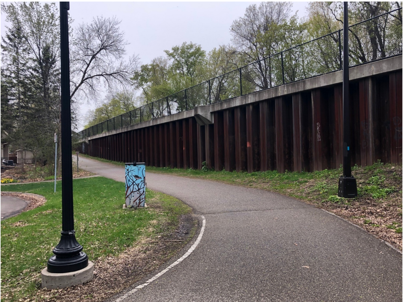
Figure 6 – Sheet Pile Wall Example
