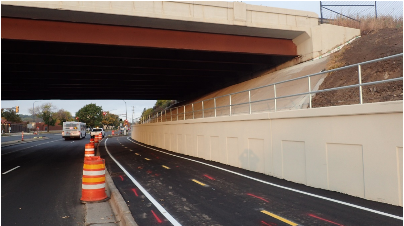
Figure 5 – Soil Nail Wall w/ Concrete Facing Example
