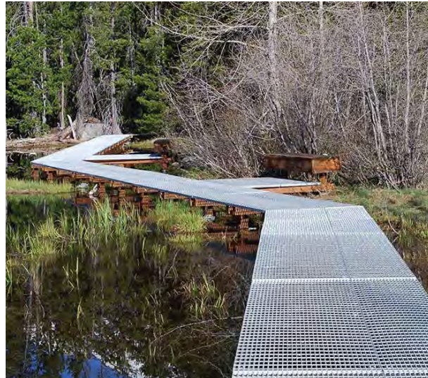
Impervious surface Removal
