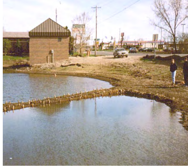
In-Lake Treatments (Permanent Structure)
