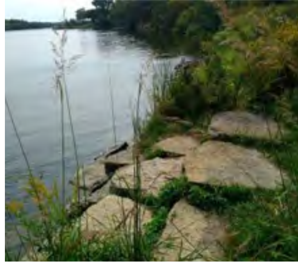
Stablized, Consolidated Lake Access Points
