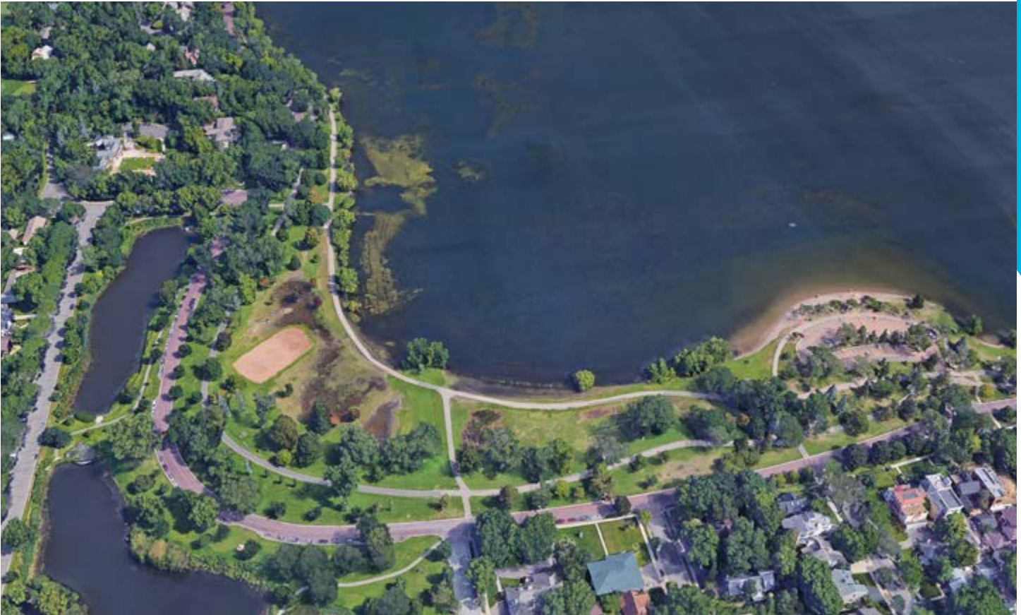
This 2014 aerial photo shows the wetland complex in the southwest corner of the lake which has been effective in improving water quality of the lake. Note the inundated recreational lawns rendered unusable by high water conditions.
