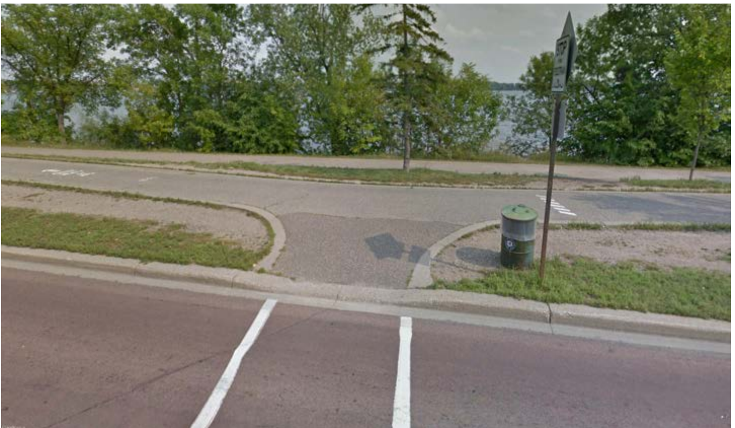
The parkway location limits recreation space and natural habitat along the lake shore. Ramps to the trails do not meet accessibility standards.
