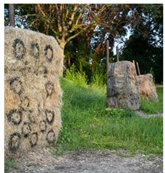
Archery facilities at William Berry Park needs significant improvements.
