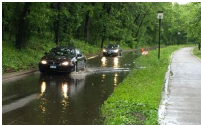
Failing storm sewer infrastructure along Lake Harriet's Lower Road leads to flooding and road closures.
