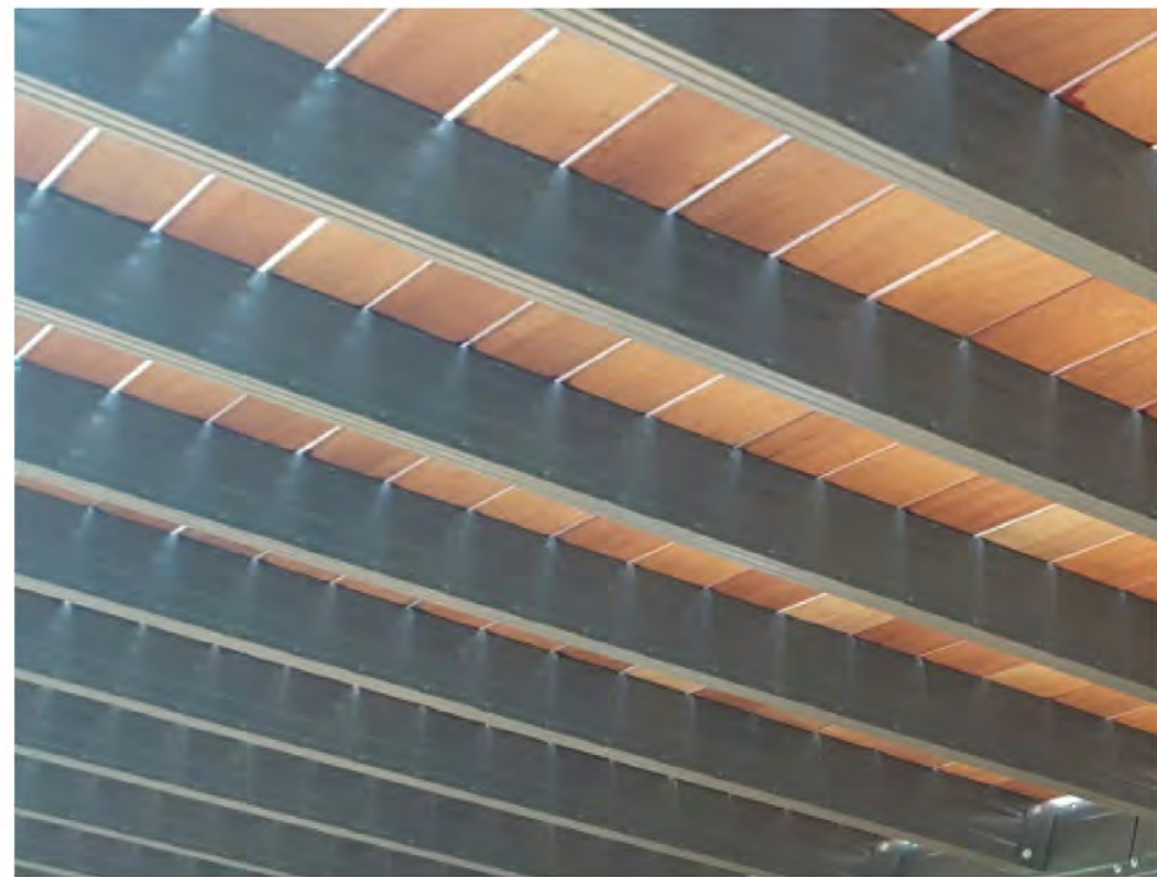
WOOD ROOF DECK STEEL ROOF STRUCTURE
