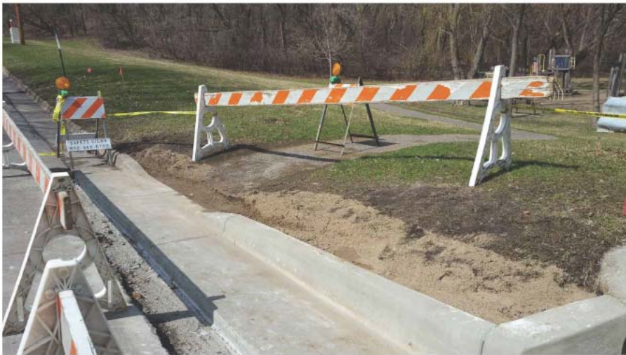
New curb ramp and storm drain
