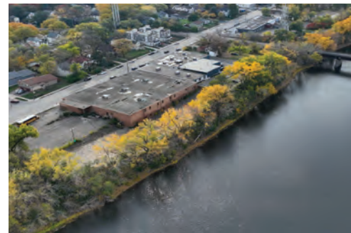
East bank at 1720 Marshall St NE
