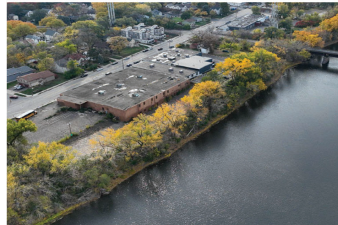
East bank at 1720 Marshall St NE
