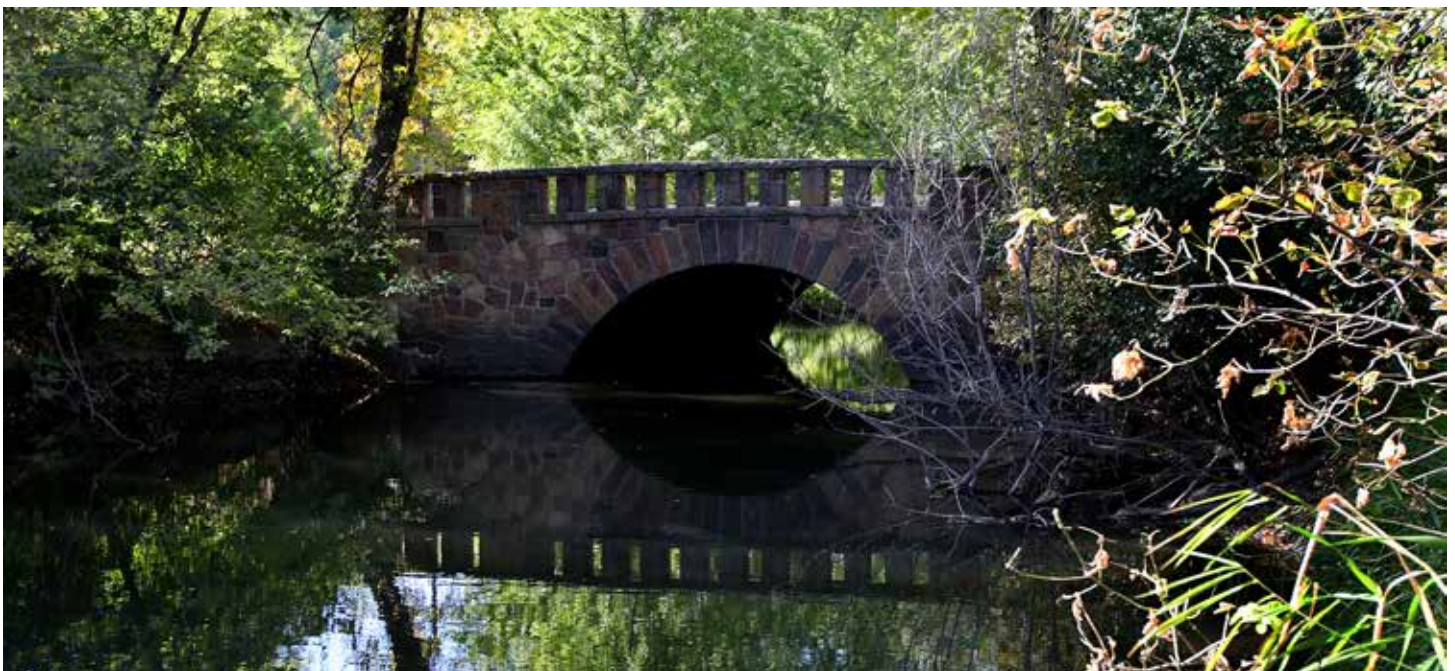
Figure 90. Bassett Creek bridge.
