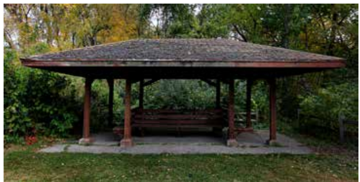
Figure 61. Glenwood Line Streetcar Shelter.
