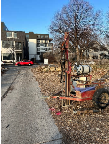
View of LGP-1 investigation location
