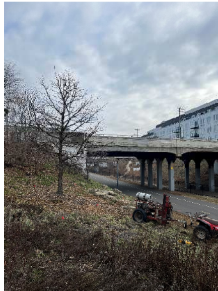
View of LGP-4 investigation location
