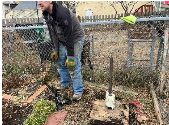
View of LGP-6 investigation location
