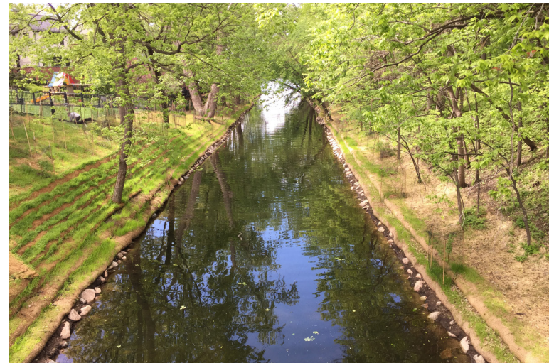
Kenilworth Channel following completion of the restoration project, 2022
