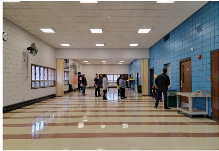
EXISTING MULTIPURPOSE ROOM
