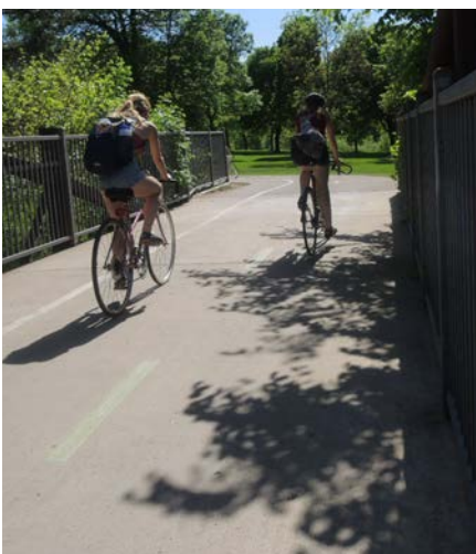
A bridge across Minnehaha Creek narrows the separation between bike and pedestrian traffic
