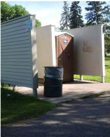
Park users identified the need for more portable restrooms throughout the park
