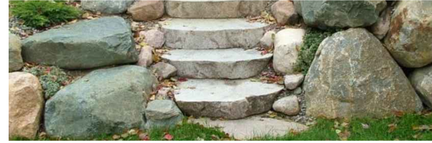
COMBINATION BOULDER WALL AND BOULDER SLABS AT UPLAND WALL
