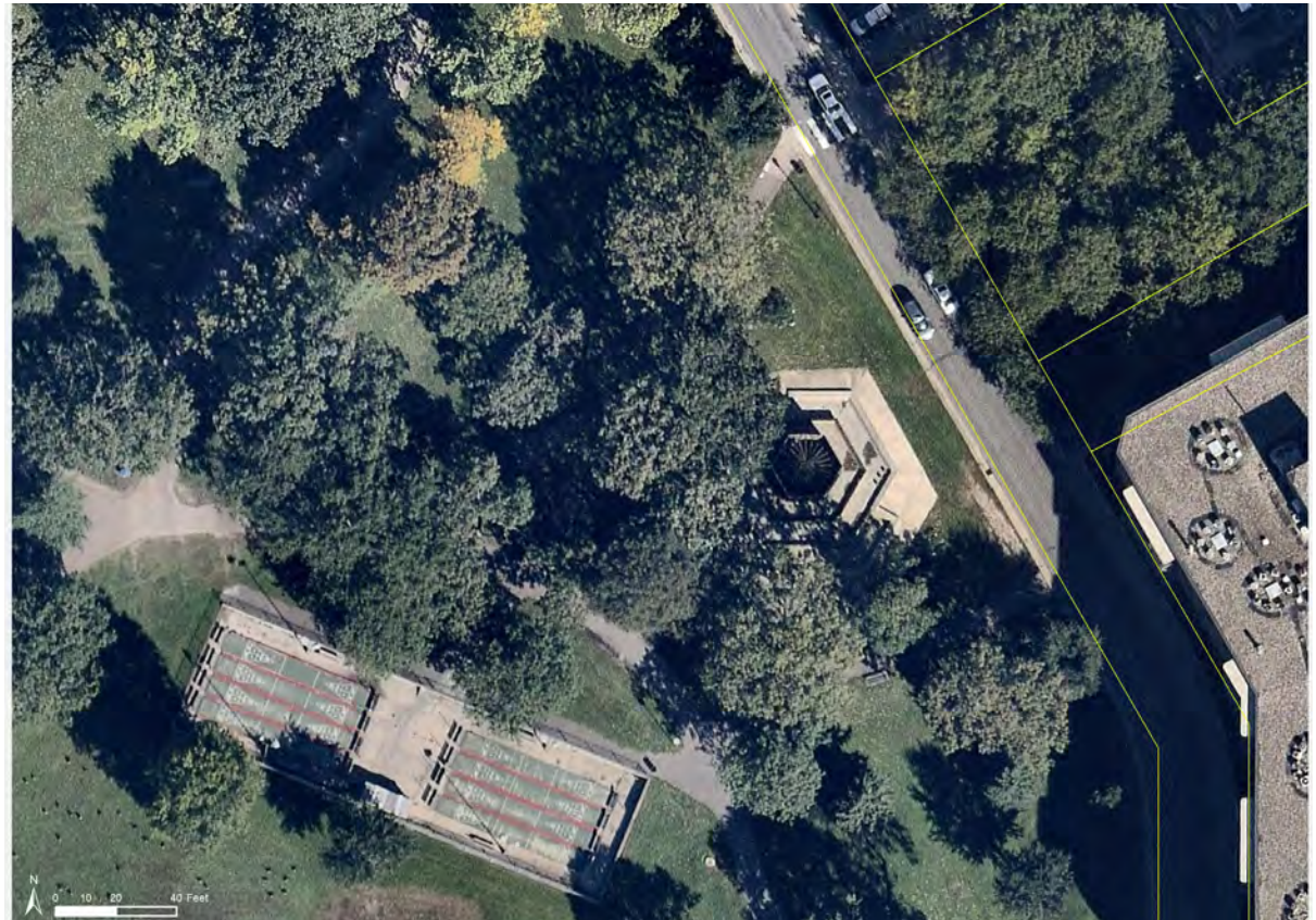
Figure 1.42 Berger Fountain Existing Conditions
