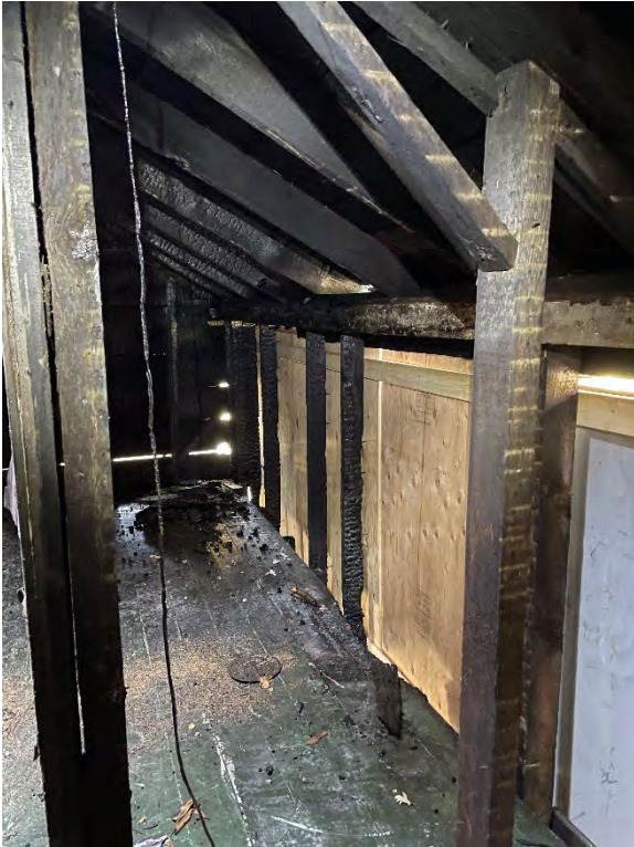
Photo 33 North chamber east elevation.
