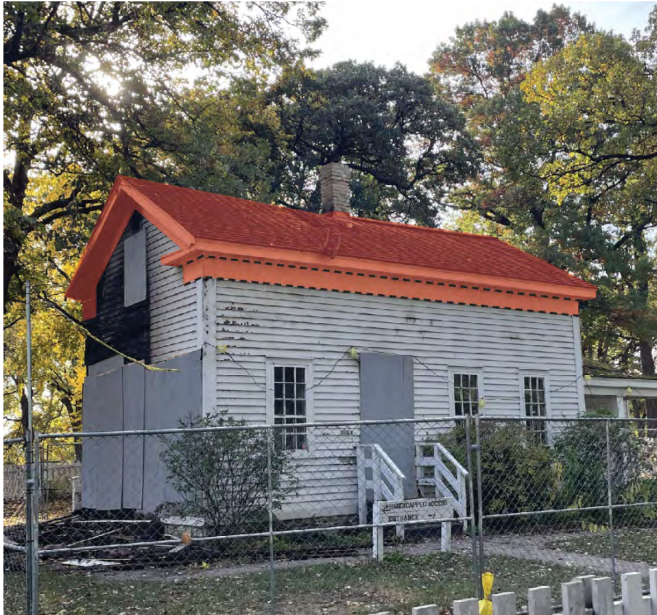
Photo 5 Northern and western facades.
