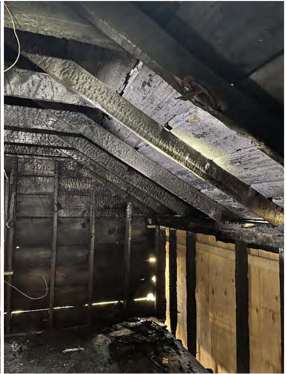
Photo 32 North chamber northeast corner.
