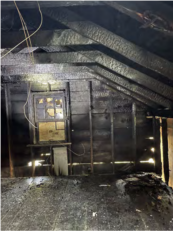
Photo 31 North chamber north elevation.
