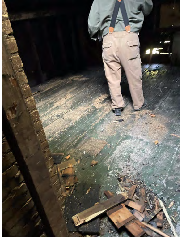
Photo 34 North chamber floor condition.
