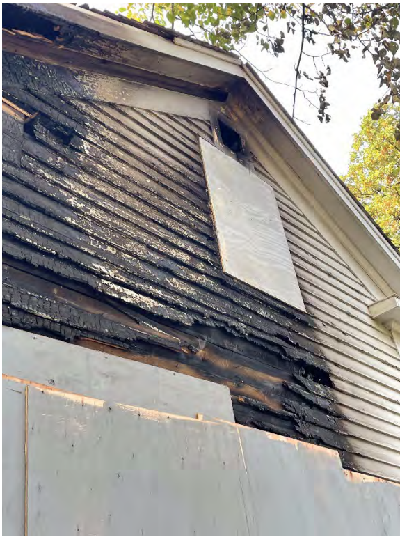
Photo 16 North 2nd floor window.
