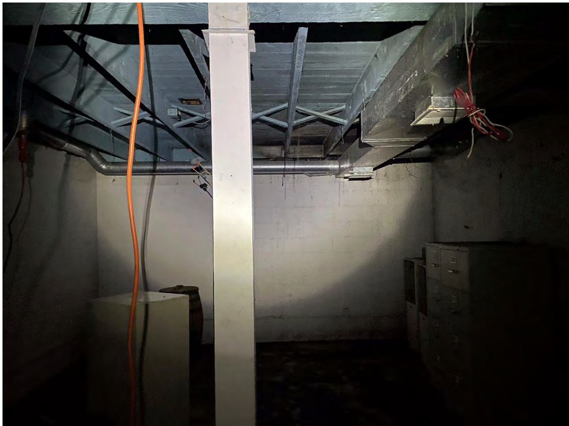
Photo 18 North elevation of basement meeting room.
