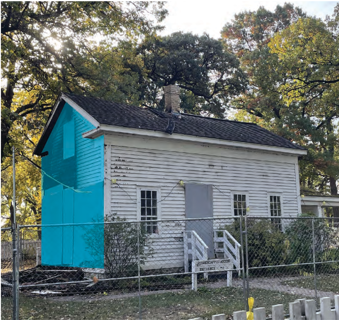
Photo 2 Northern and western facades.
