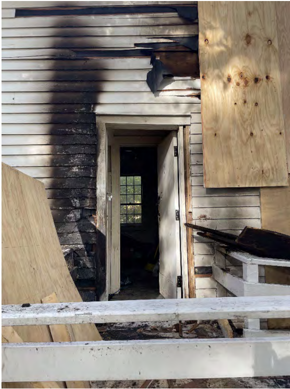
Photo 14 East entry door.
