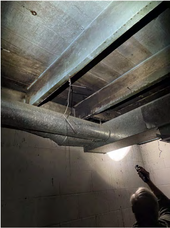
Photo 19 NE corner of basement meeting room.
