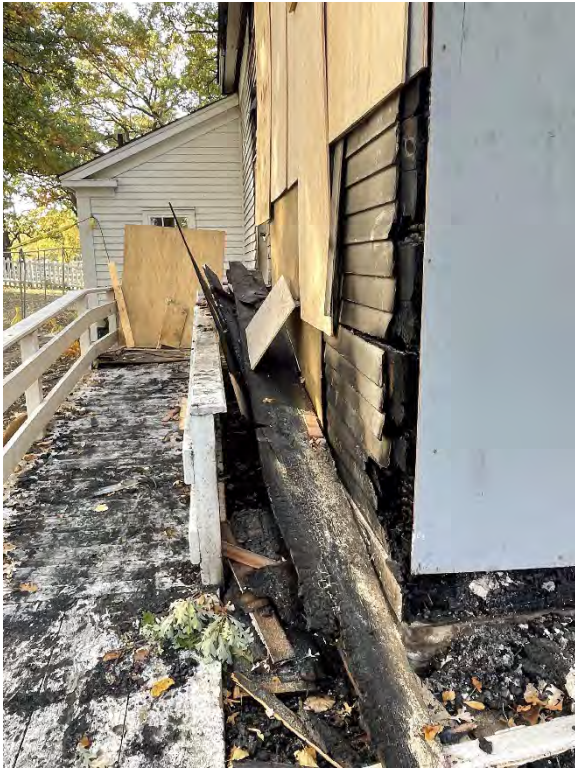
Photo 12 East elevation, looking south.
