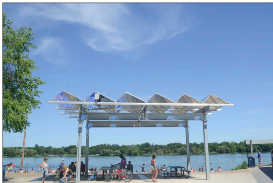
Nokomis Main Beach solar shade
