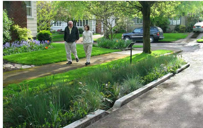
Bioswale in planting strip
