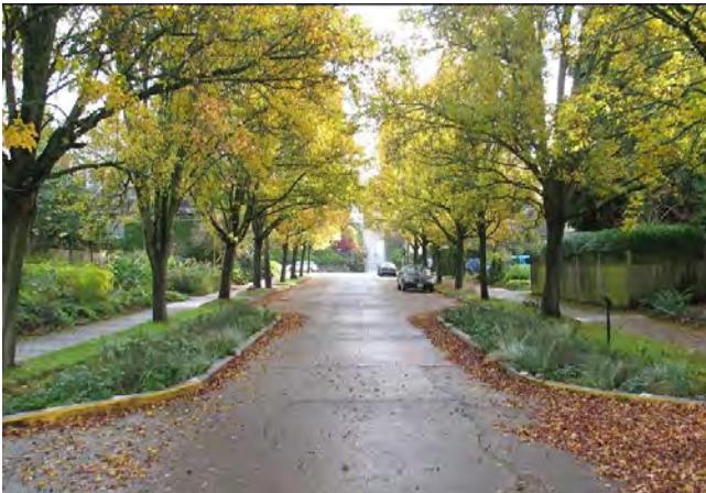
Bioswale in curb extensions
