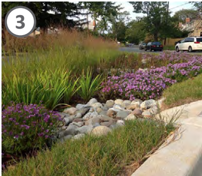
3 Stormwater / Rain Garden
