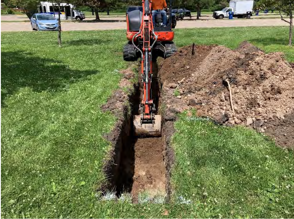
Photo 7: TE-04-20, facing north
