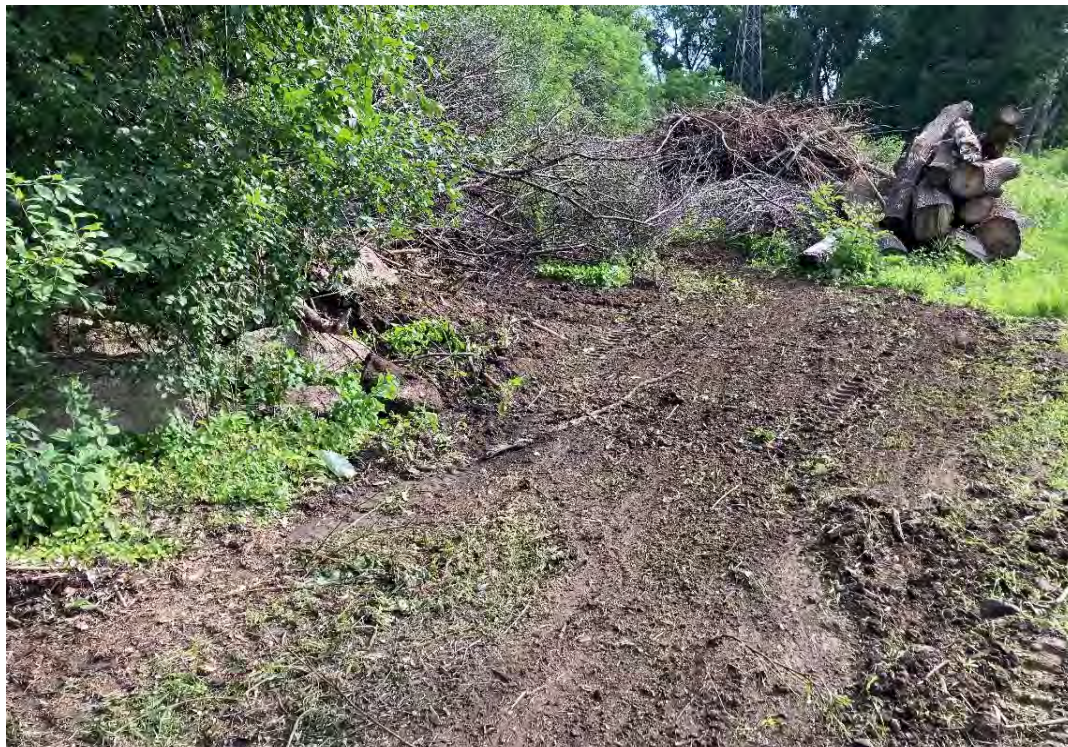
Photo 14: TE-09-20, backfilled; concrete debris observed on ground surface
