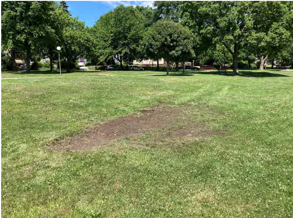
Photo 6: TE-03-20, backfilled and seeded
