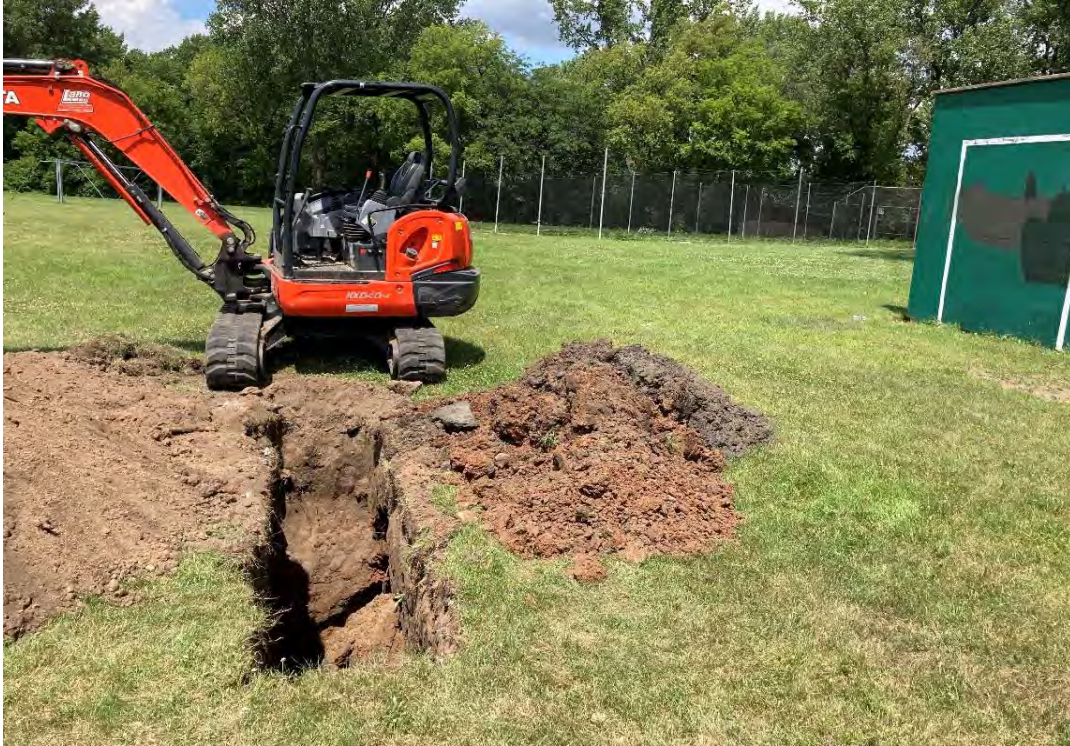
Photo 21: TE-14-20, facing north
