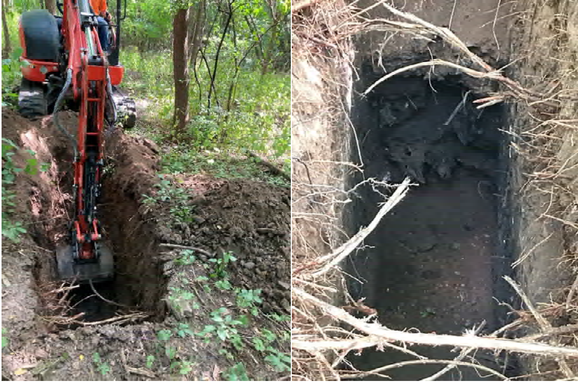
Photo 9a: TE-06-20, facing south
