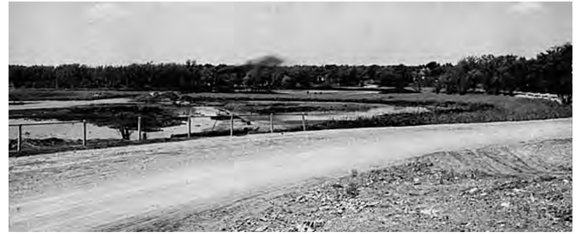
Dredging Lake of the Isles - 1909
