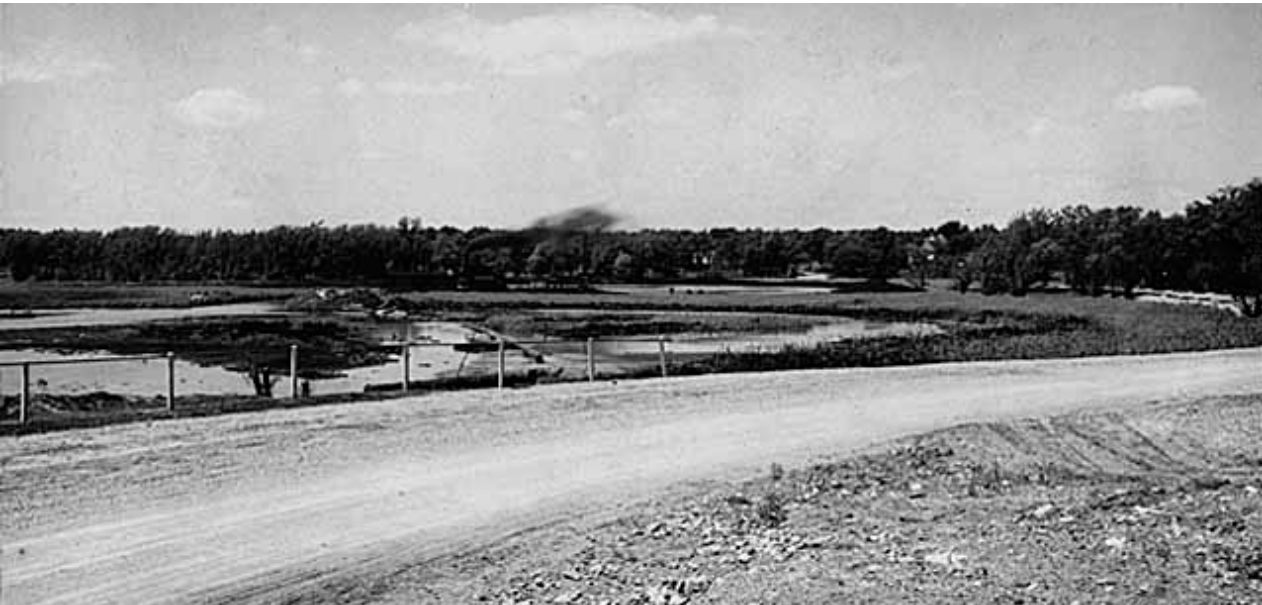
Dredging Lake of the Isles - 1909
