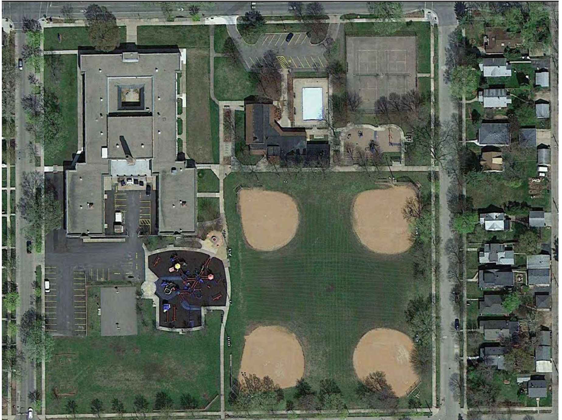
Existing Conditions: Hiawatha School
